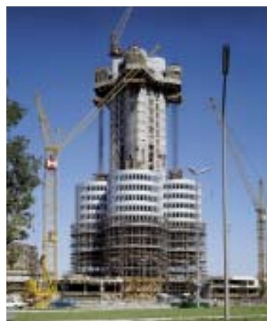
Top | View of the BMW Tower from the Olympic Stadium during the Olympic Games.
