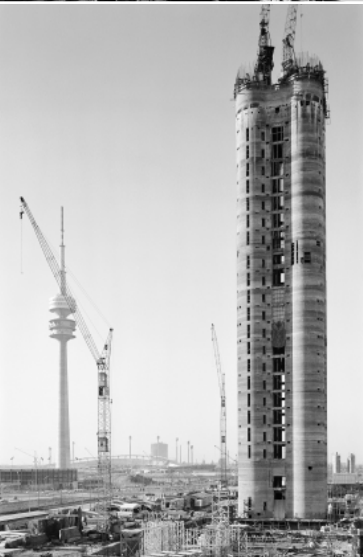
Top | The first seven storey segments are raised with the assistance of the technical storey below (optical waistline) and a special cable construction.
