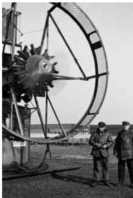
Left: Cutaway of the BMW 132 A aero-engine in 1933, the most successful radial engine of the 1930s. Right: The Hornet engine passes its sampling test in Berlin, 1930.
